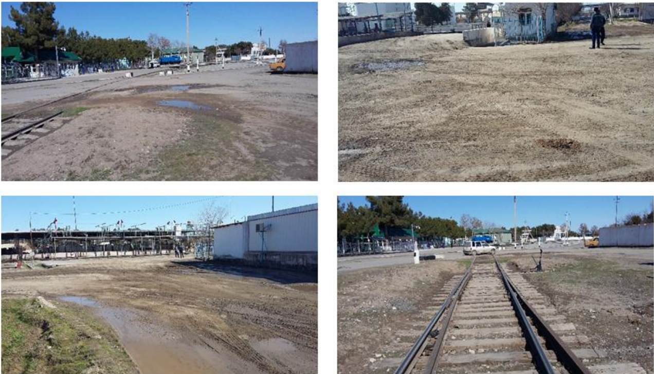
Figure 3 Road conditions at Jarqorgonneft JSC beyond the boundaries
